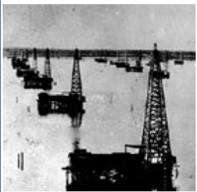
Platforms enable drilling of first submerged wells
